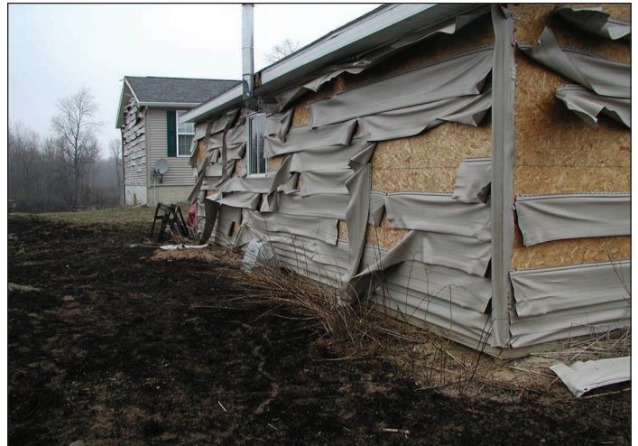
Figure 4. A wildfire in a grassy field melted the siding on this garage and home.
